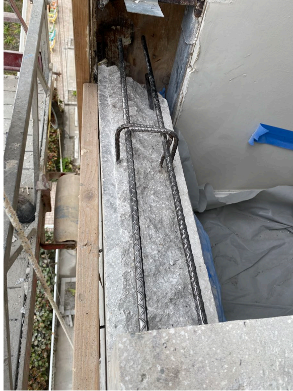
Picture 1: Unit 505 window sill repair
